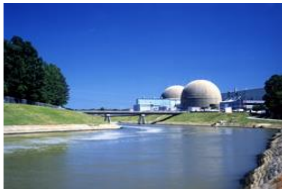
Surry Power Station
