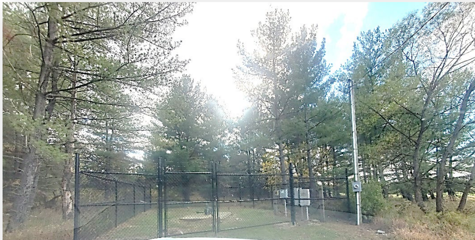
Well Fencing- Purcellville
